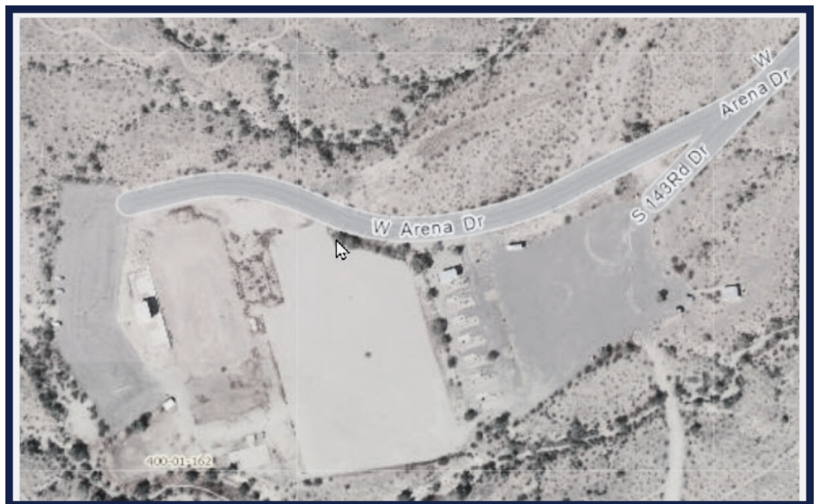
Area prior to improvements.
